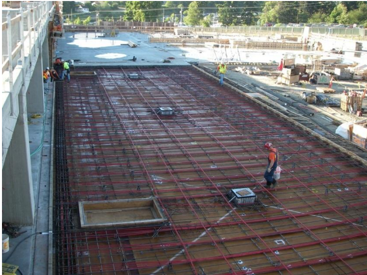
QTA #4 Post Tensioned Deck Installation
