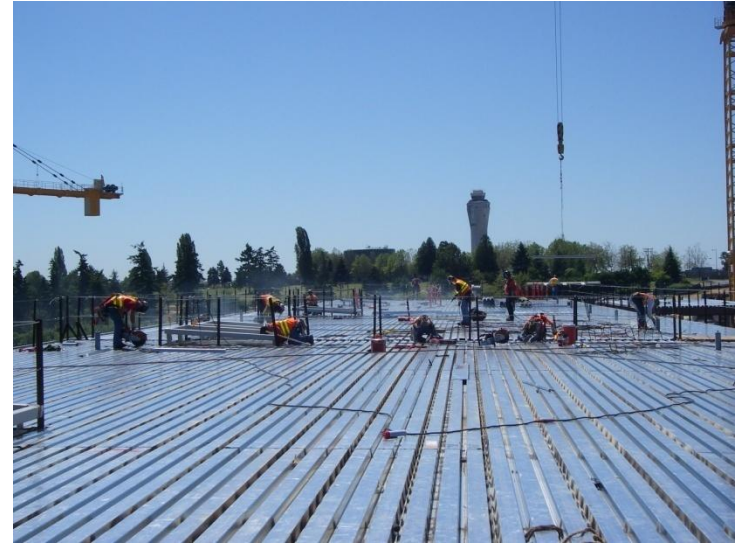
Metal Deck Installation on East High Roof
