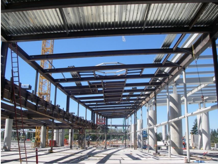
Customer Service Building & High Roof Progress
